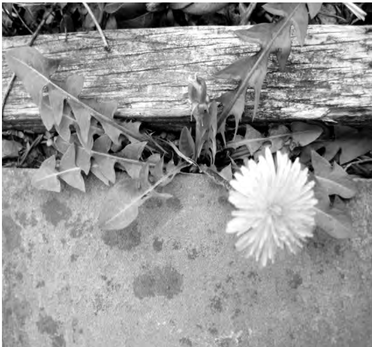
Dandelion growing in the crack of the sidewalk.
